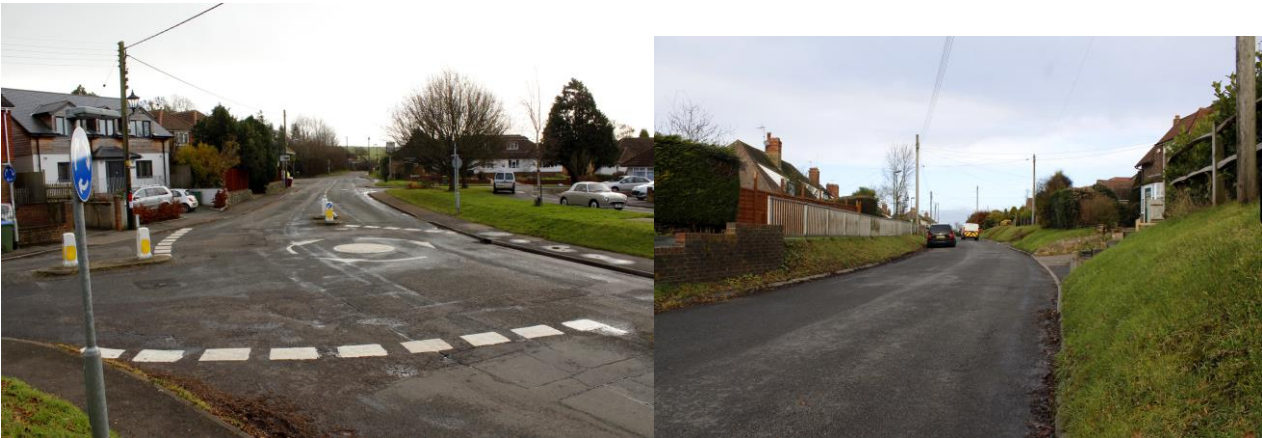
Poor Road layout and Narrow width leads to problems in peak periods
