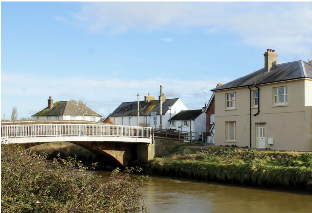
The Old Bridge with new footpath added
