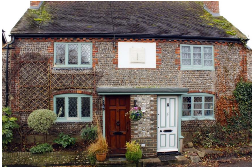
Hyde lane Cottages with Flint Frontage
